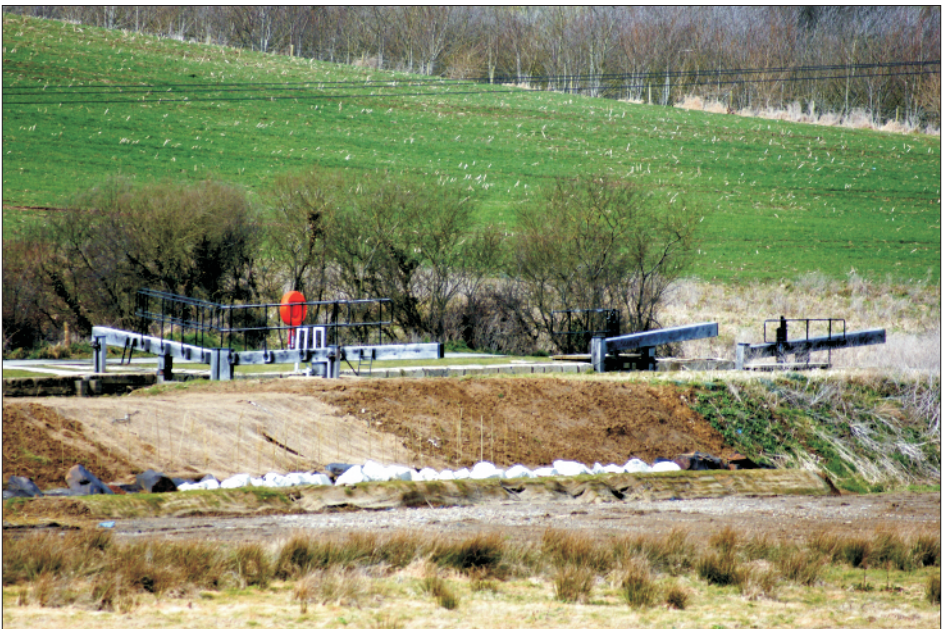
Whalesborough Lock showing new spillway Photo: Mike Moore
